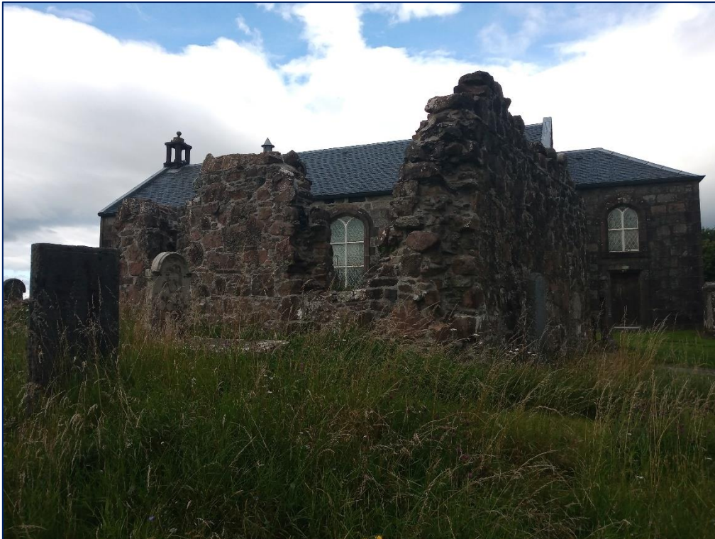
Plate 7.39: North facing view of the Scheduled Old Parish Church of Muckairn (Asset 42) with the existing Church in the background
