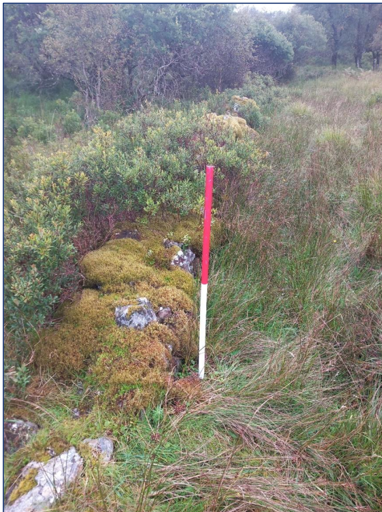
Plate 7.3: North facing view of a section of stone built wall (Asset 139) within the Site
