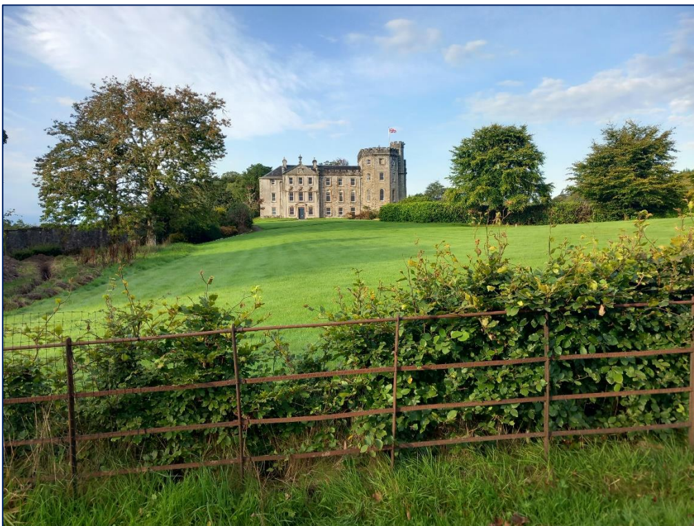
Plate 7.17: South-west facing view towards Lochnell House, Ardmucknish Bay (Asset 88)
