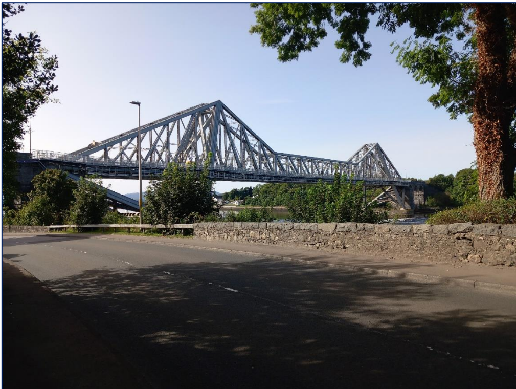
Plate 7.48: East facing view of the Category B Listed Connel Ferry Bridge (Asset 100)
