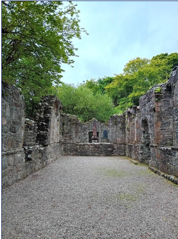
Plate 32: View of Dunstaffnage Castle Chapel (Asset 18)
